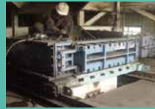
On-site Repair of Model 500 Crusher
